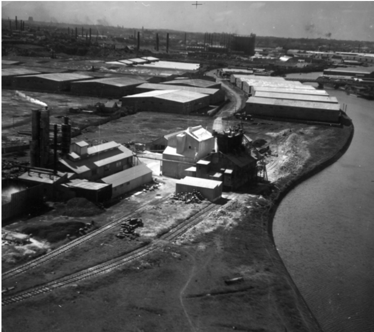
Figure 83: (Left) Oblique aerial view of the lime burning plant on Alexandra Canal, not dated (late 1940s). Looking north with Burrows Road and adjoining wool stores in the background. Source: Royal Australian Historical Society (21841032)
