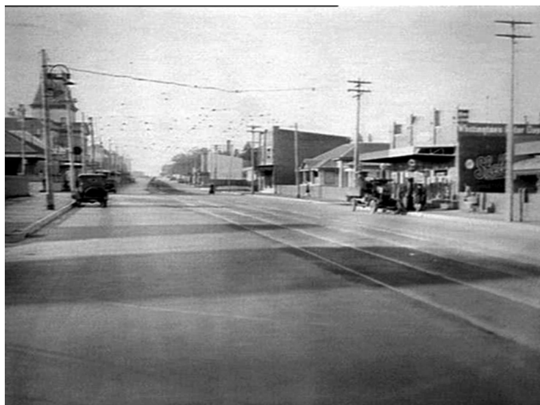
Figure 87: (Left) Princes Highway from Gannon Street, Tempe, with the ornate cupola of the Pulteney Hotel (now Tempe). Dated July 1928 and prior to alterations. Source: State Library of New South Wales (Government Printing Office 1-13131)
