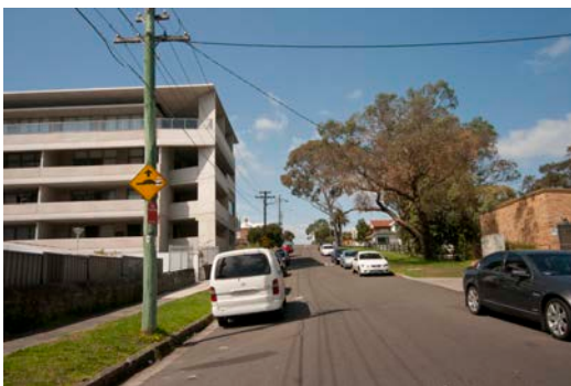
Figure 134: Residential flat building in Thornley Street, Marrickville (Sub Area 4)
