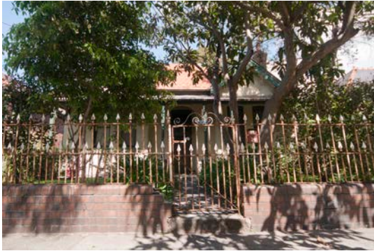
Figure 149: Cement rendered Federation Queen Anne style house at No. 24 Silver Street St Peters (Sub Area 6)
