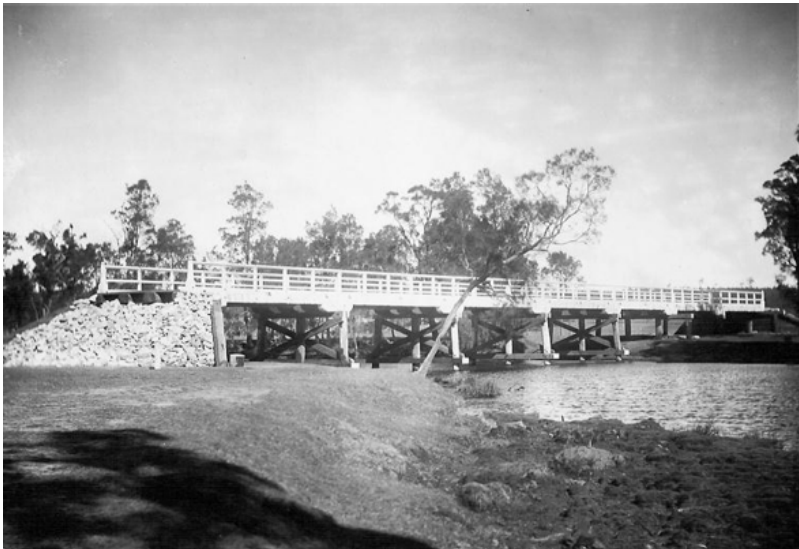
Figure 97: (Left) The former timber bridge of the crossing of Cooks River at Wardell Road in 1911. The bridge, pictured while under construction, was replaced by the existing reinforced concrete bridge in 1924. Source: Souvenir to commemorate the 50th anniversary of the incorporation of the Municipality of Marrickville , Marrickville Municipal Council, 1911
