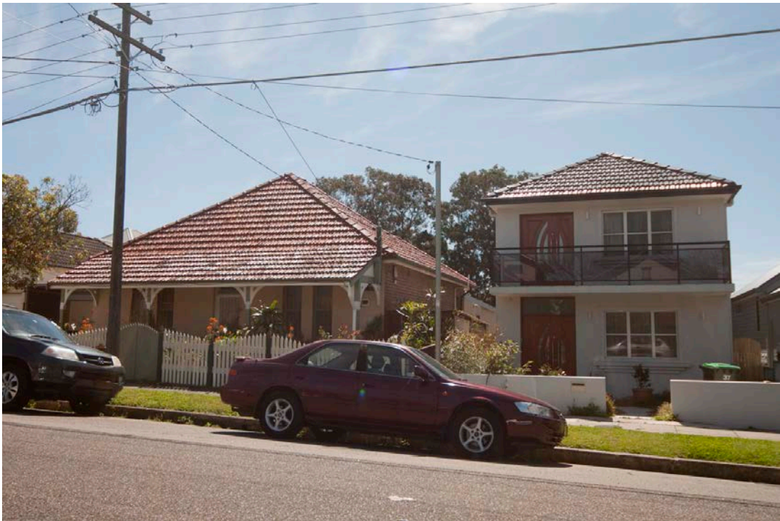
Figure 130: Old and new housing adjacent in Cary Street Marrickville (Sub Area 4)
