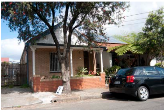
Figure 147: An older house reclad in circa 1970s brickwork, with aluminium framed windows in Grove Street St Peters (Sub Area 6)
