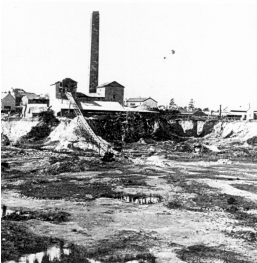
Figure 41: Ernest Loftus Speare's Tempe Brick, Tile and Pipe Works c.1935 on the Princes Highway south of Bellevue Street. This photograph is usually reproduced as being of Goodsell's pit behind May Street, but appears to be the Tempe Brick, Tile and Pipe Works. Source: Ringer, Ron, The Brickmakers 1788-2008 , Dry Press Publishing, 2008, p.168
