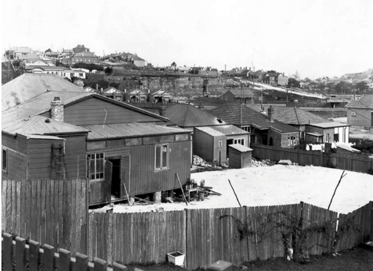
Figure 46: (Left) In the background is George Schwebel's quarry beside Illawarra Road in 1936. Source: Marrickville Image Library (000894)
