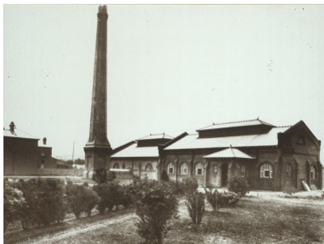
Figure 60: (Left) A photograph of the Marrickville Pumping Station taken in 1897 Source: Local Studies collection, Marrickville Council Library
