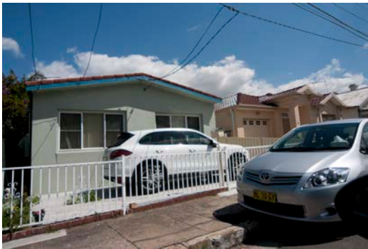
Figure 161: Circa 1960s and modern housing, Wentworth Street, Tempe (Sub Area 10)
