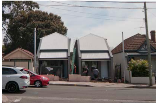
Figure 144: New townhouses under construction in Unwins Bridge Road (Sub Area 5)
