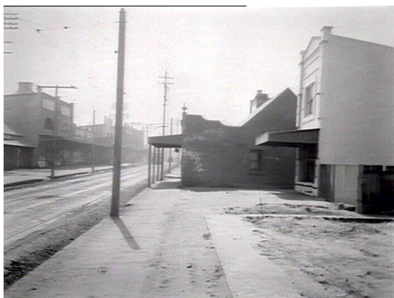
Figure 99: The old and new building alignments of Princes Highway, September 1926. Source: State Library of New South Wales (Government Printing Office 1-12704)
