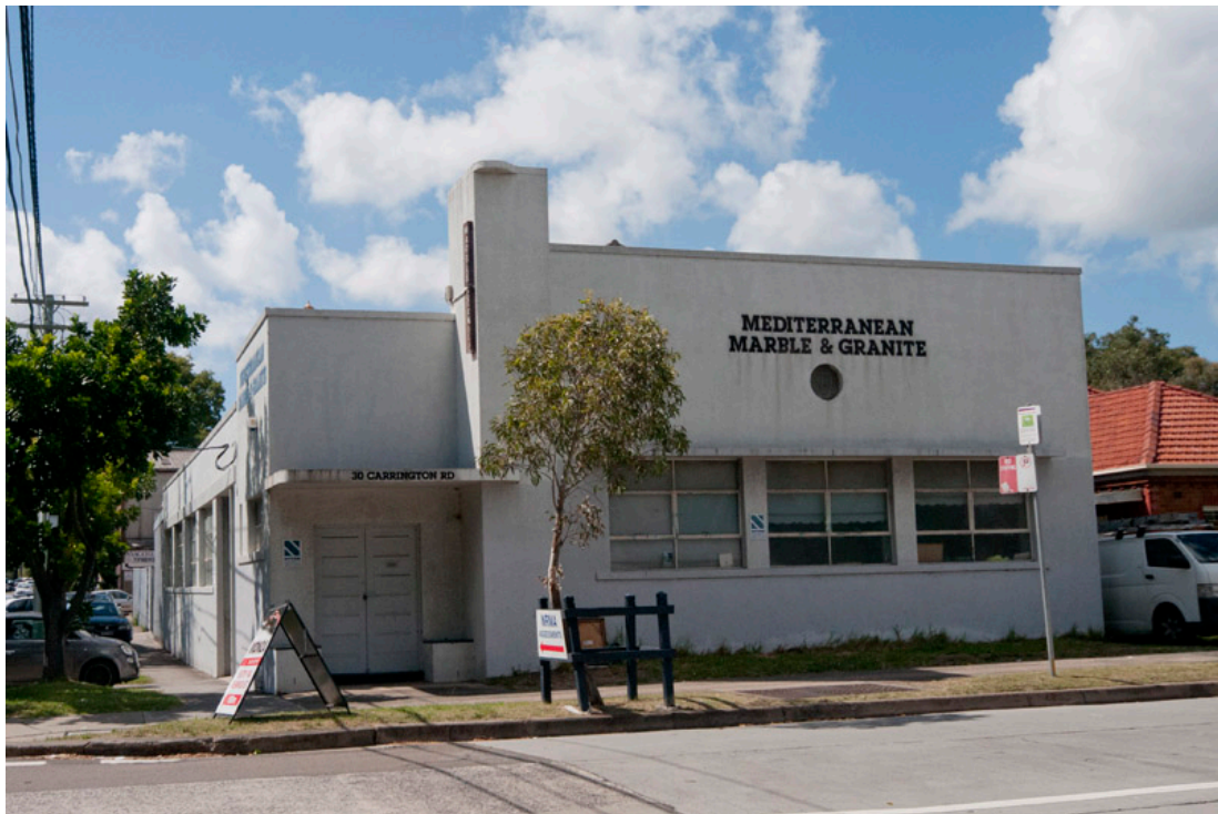
Figure 117: No. 30 Carrington Road (corner Renwick Street). This factory building was constructed in 1949
