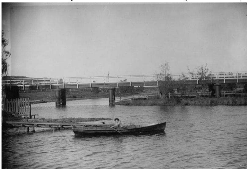
Figure 95: The old timber bridge erected by PA Tompson and the government's then modern iron bridge on Cooks River at Illwarra Road. Parts of the iron bridge remain. Source: Australian Town and Country Journal, 3 /4/1880, p.24
