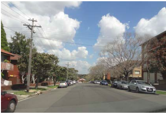
Figure 120: 1970s residential flat buildings in Bayley Street, Marrickville (Sub Area 2)
