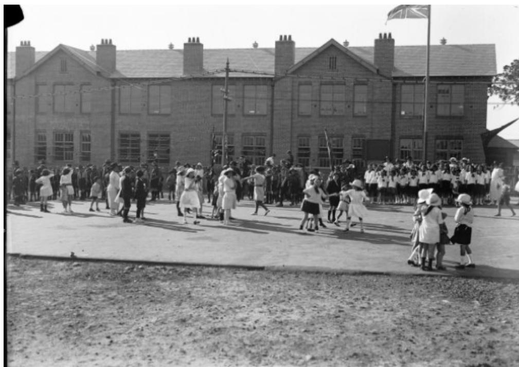
Figure 110: Tempe public school. Not dated. Source: National Library of Australia (pic-vn3098407-v)
