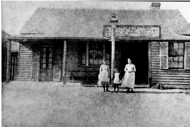
Figure 88: (Left) Cottage of Content Hotel at Tempe (later Riverview) prior to rebuilding around 1892. Not dated (c.1892). Source: Marrickville Image Library (003222)
