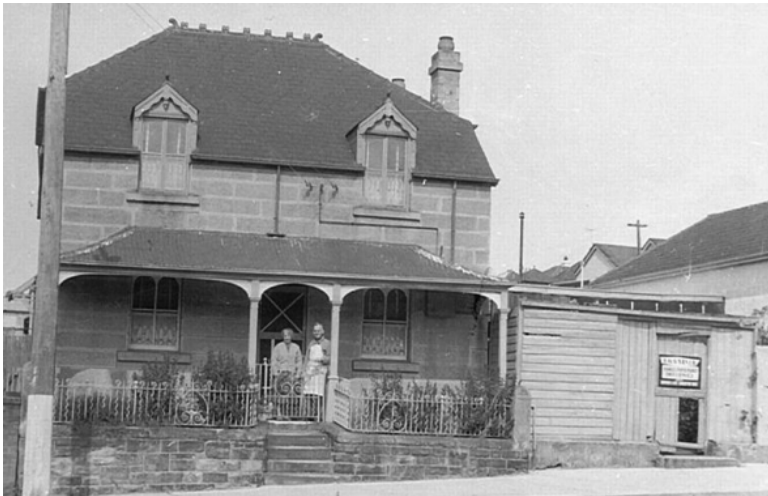
Figure 45: (Left) The former home of Adam Schwebel in Illawarra Road out of stone quarried from their yard at Schwebel Street. Demolished in 1965 and the stone was used in the boundary wall of Roseby Memorial Church. Source: Marrickville Image Library (001833)
