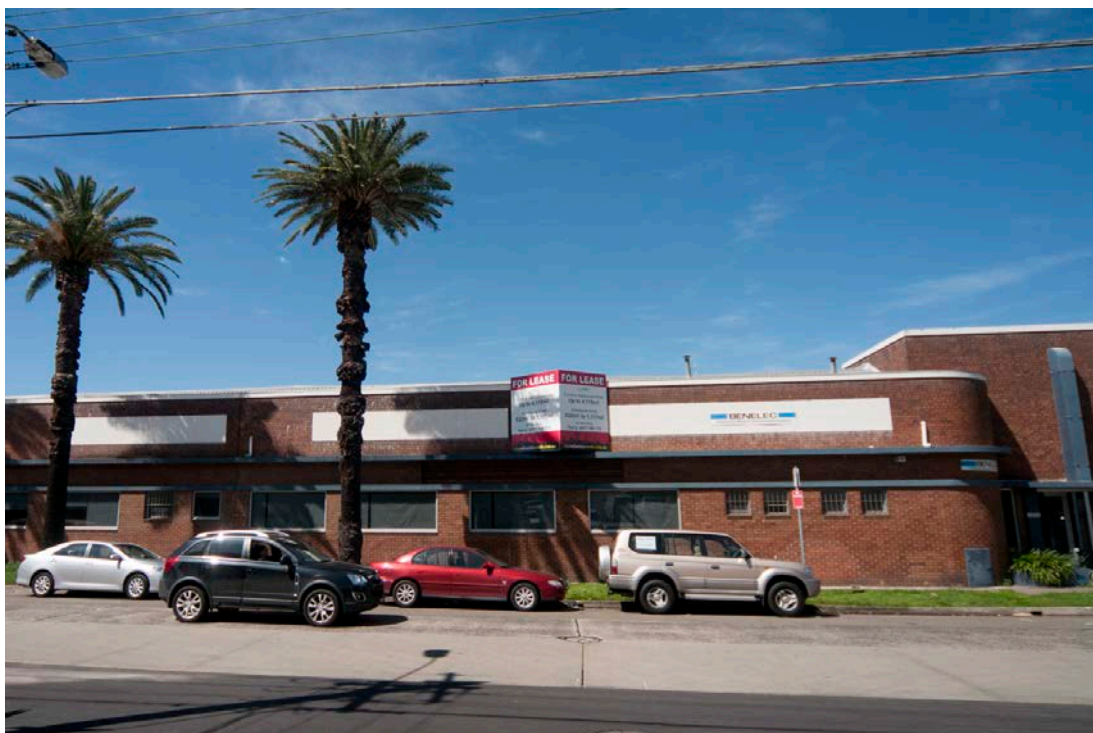
Figure 115: No. 6 Carrington Road, Marrickville – formerly extended storage and factory floorspace for General Motors Holden. The building dates to prior to 1939 (appears on 1943 aerial photo)
